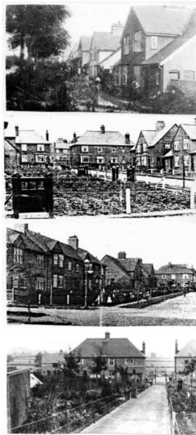
Figure 31 (a) – Humberstone Garden Suburb Houses 1907-1914 (from The Link)
