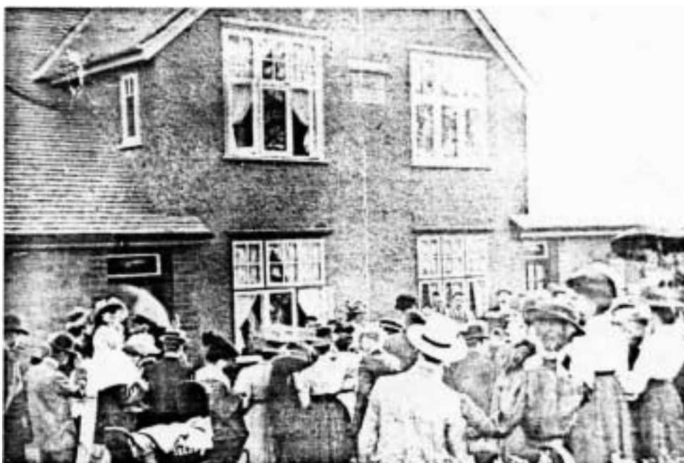
Figure 9 – Formal opening of the first pair of cottages, October 1908
