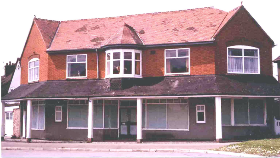
The Laburnum Road shops
