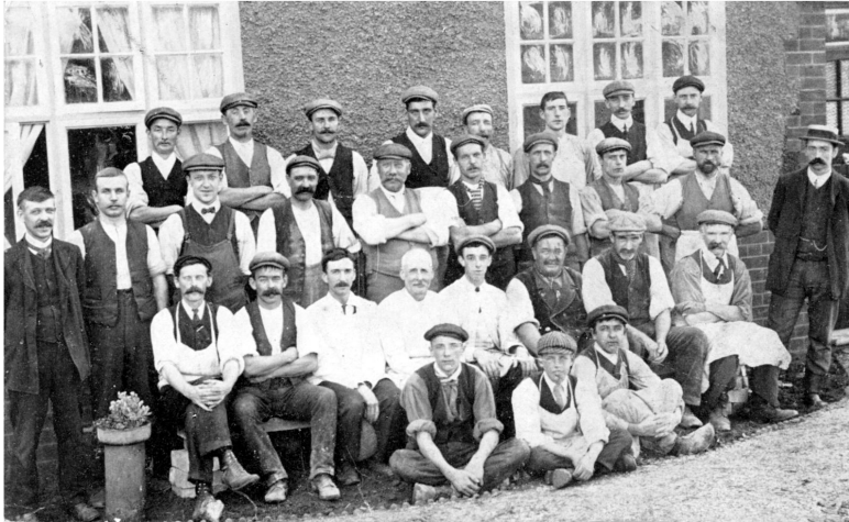
The builders - November 1908
